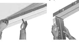
Sleeve the hinge jamb over the wall. Bring the header down tight, interlocking the stop in the alignmenttab. **Try to** place the hinge jamb close to the stud to assure more room for adjustment in future steps.
