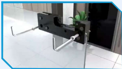
INSTALL GLASS TOP PATCH
